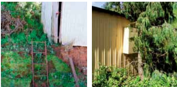
Examples of unsafe access.
