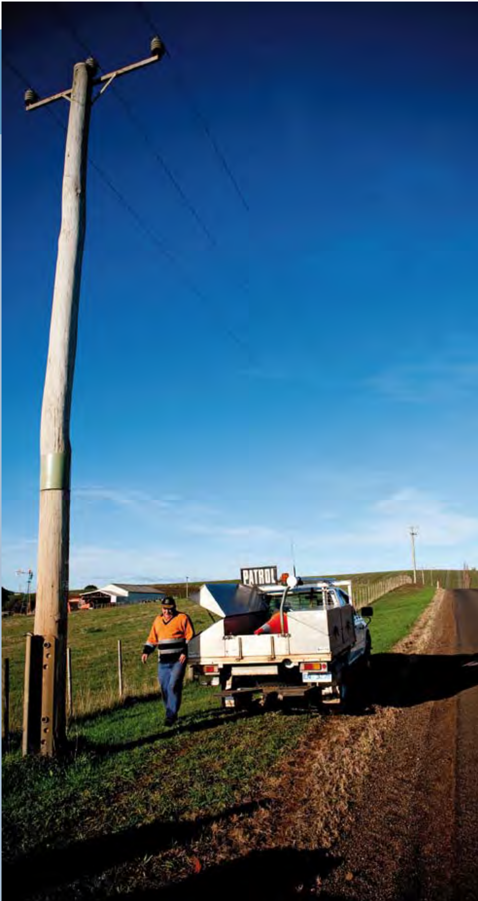
Asset inspector Case Van Tatenhove on his pole inspection round south of Latrobe. Aurora spent $10.3 million inspecting and maintaining poles this year, to protect the safety of our system and our customers.
