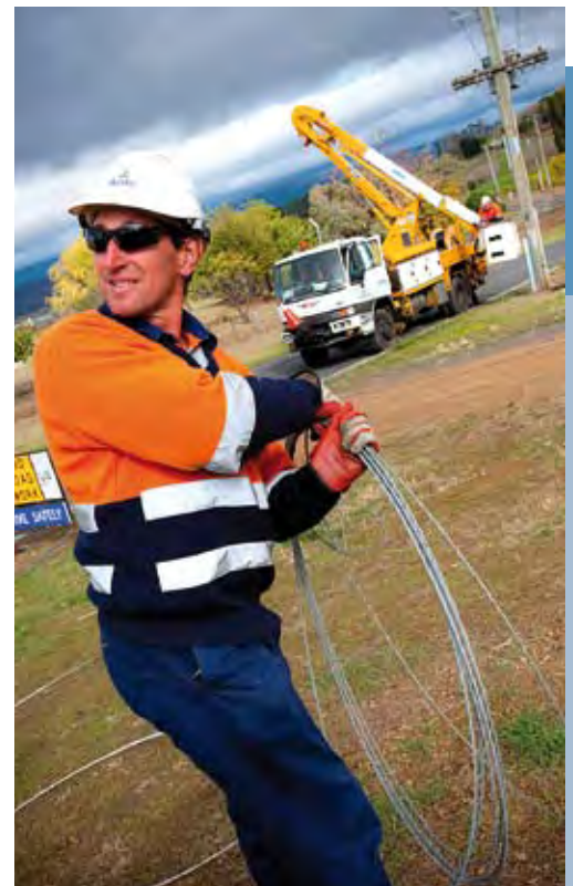
Lineworker Rodney Cowle.
