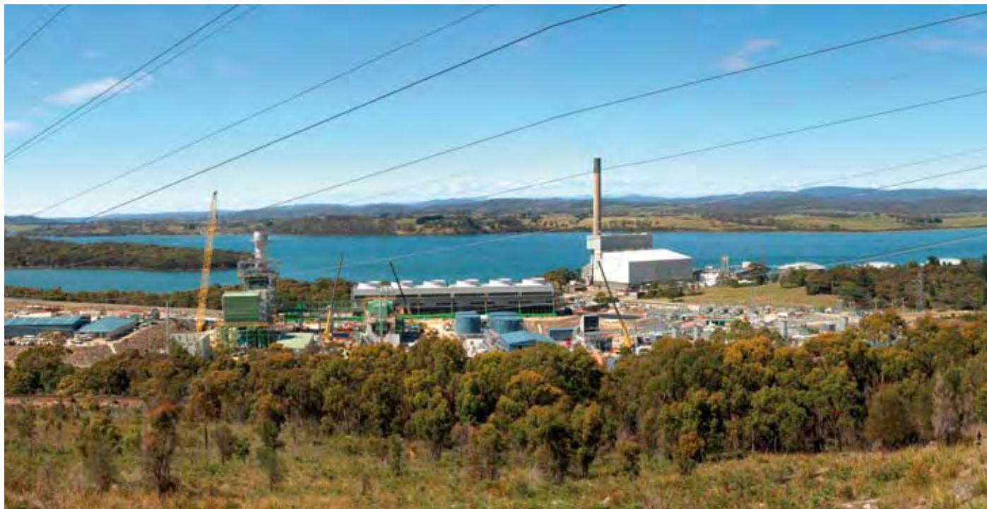
Construction under way at the Tamar Valley Power Station.
